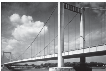
Fig. 2: Suspension Bridge across River Rhine at Köln, Germany (1938–1941), main span 378 m
